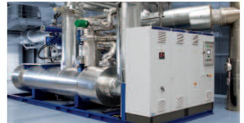
Dürr’s Cyplan 70 kW compact module generates electricity from waste heat.
